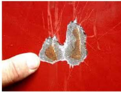
Due to corrosion
